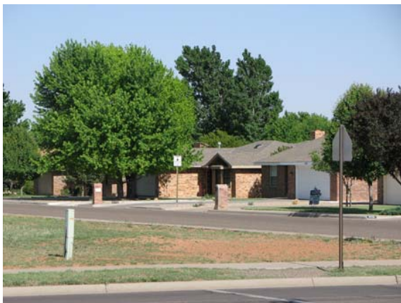
Photo 2-4 Existing neighborhood in Clovis
