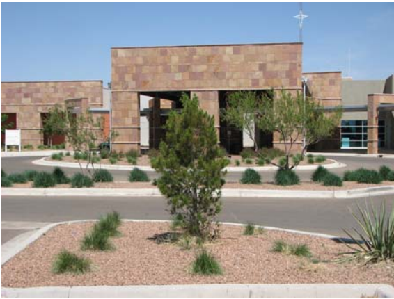
Photo 3-7 Clovis - Plains Regional Medical Center Emergency Facility
