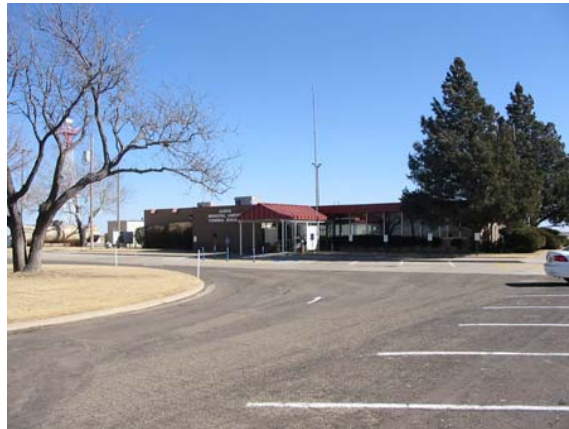
Photo 2-13 Clovis Municipal Airport Terminal Complex
