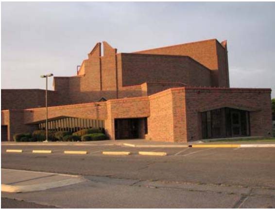
Photo 5-5 ENMU performing arts facility
