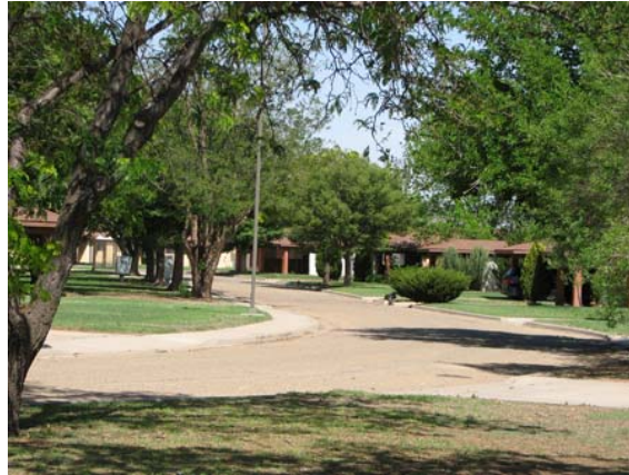
Photo 2-1 Chavez West 801 Housing in Clovis
