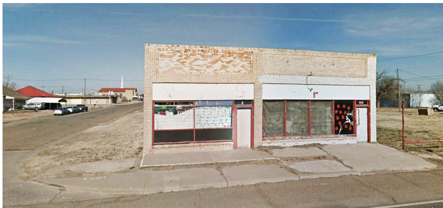
Top: Intersection at 2nd Street and Alphon Street in MRA District 1 - no handicapped ramps or sidewalks means that wheelchair users are in the street travel lanes. This intersection was determined to be a "low priority" for ADA improvements. Bottom: Commercial building at the northeast corner of 1st Street and Giddings Street - sidewalks are missing or in poor condition and no handicapped ramps.
