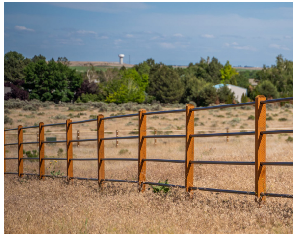
Steel pipe fence
