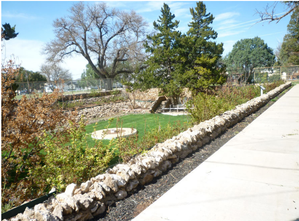
Walkway along drainage facility at Hillcrest Park.
