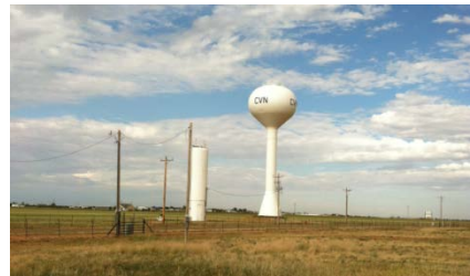
CVN Water Tower
