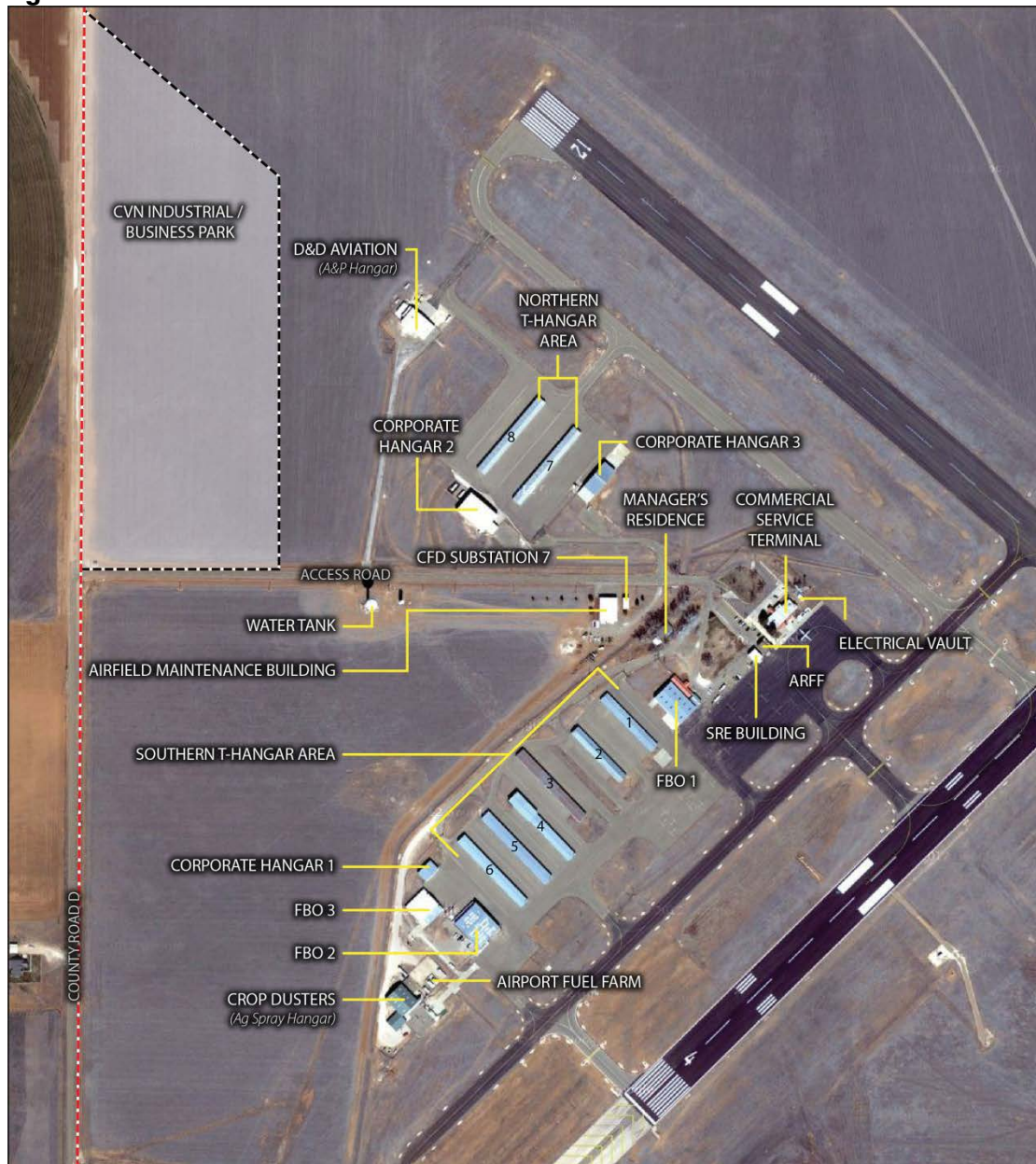
Figure 1-6: CVN Landside Facilities
